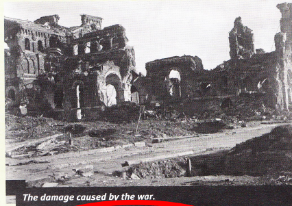
The damage caused by the war.
