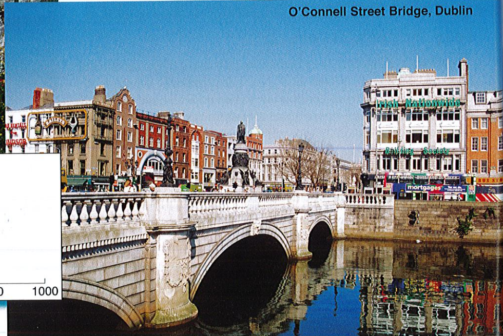
O'Connell Street Bridge, Dublin
