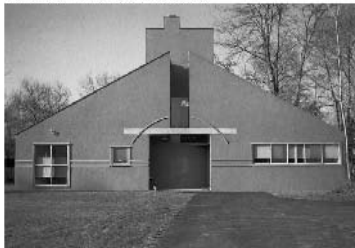
1962 Vanna Venturi House, Philadelphia, Pennsylvania, USA
