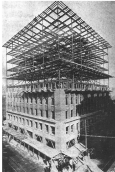
Adler & Sullivan's Wainwright "Skyscraper" building under construction (circa 1889)
